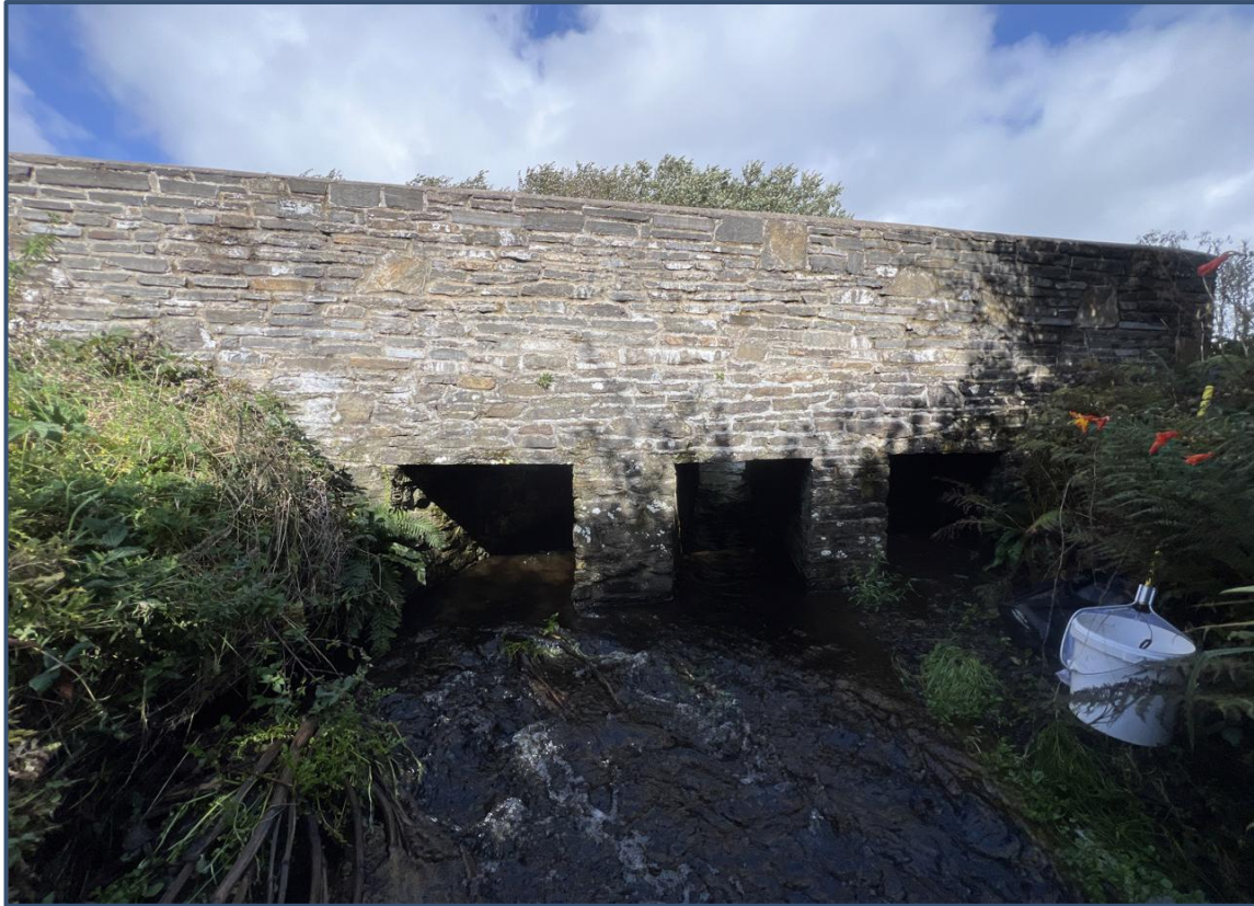
Plate 4-9. Culverted section of the watercourse where it passed under a roadbridge in the mid-section of Site WF5.
